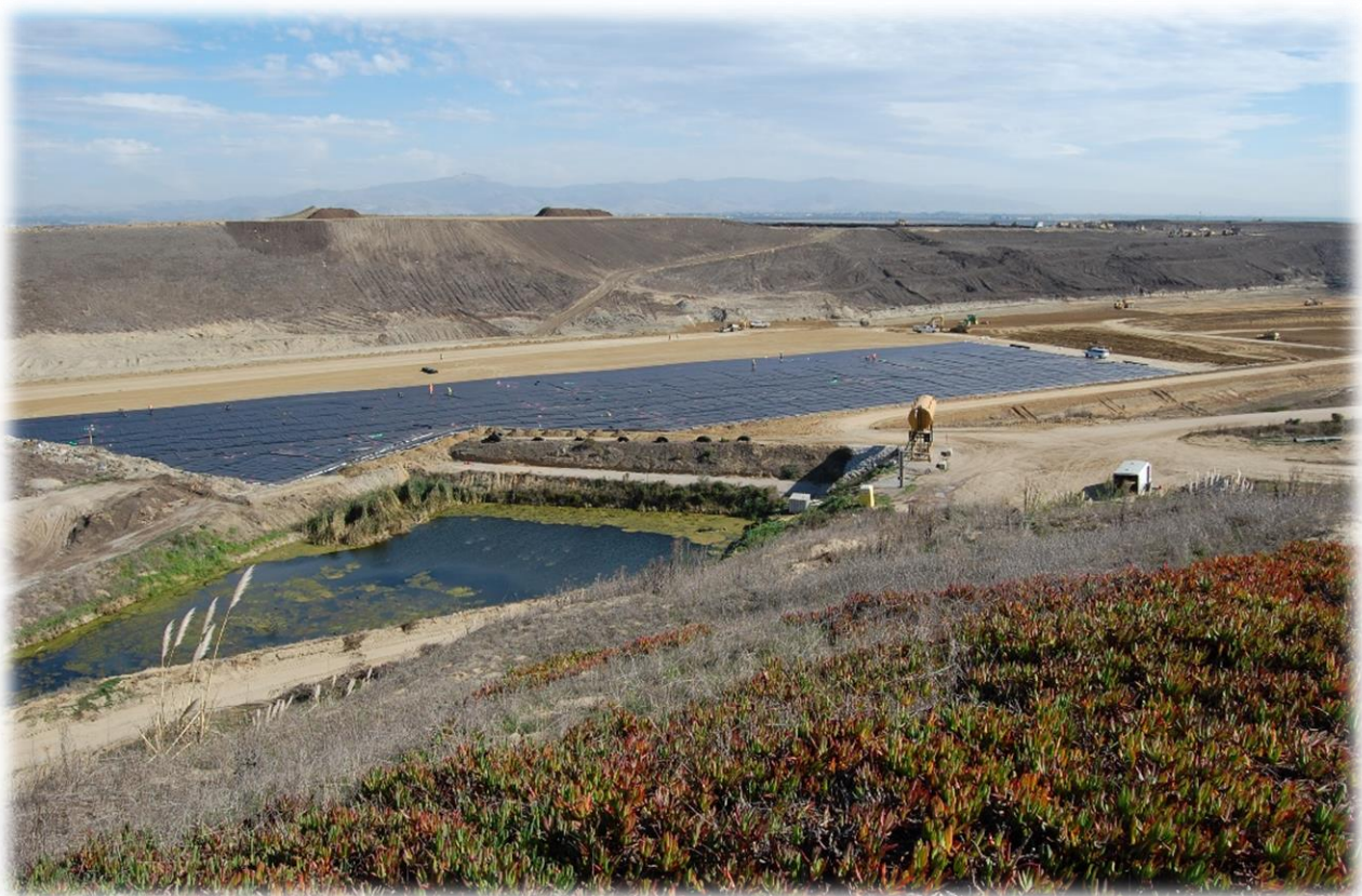
Module 5 Liner Installation
