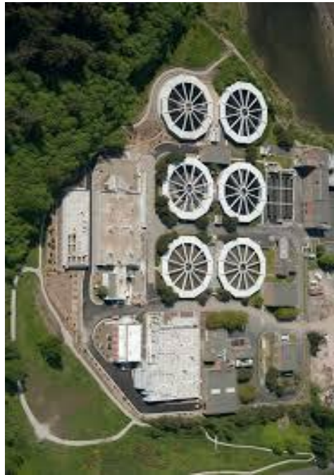
Waste Water Treatment Plant
