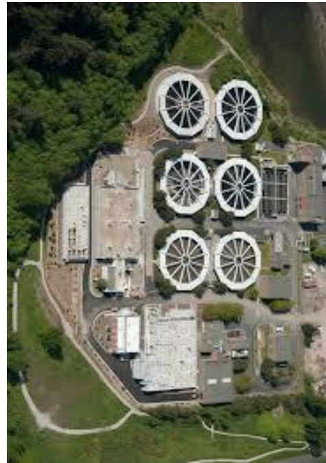
Waste Water Treatment Plant
