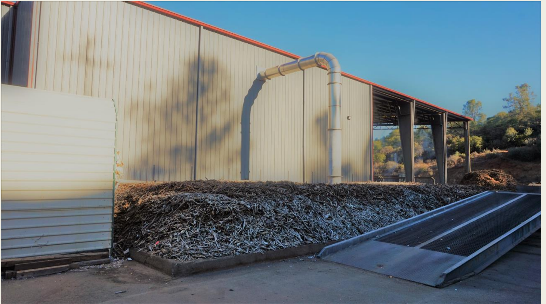
Biofiltration of the air to scrub odors
