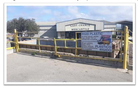
railings is installed on the top of the retaining wall between the roadway and the dumpsters to protect against falls. The setup is shown in the photo image to the left.
