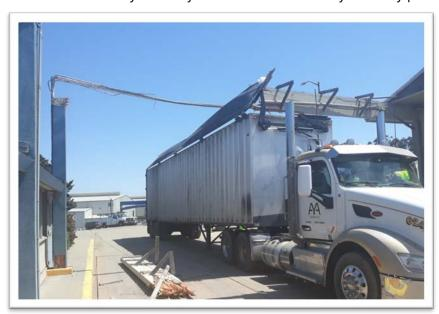
connectivity from the Administration Building to the Scalehouse. Since its construction, the Scalehouse canopies have been struck several times by overheight vehicles that have neglected to lower parts of their disposal equipment. The list of objects that have struck the canopy have included raised dumpster forks, raised payload beds, and a raised load tarp arm. The latest strikes occurred in 2018, 2020, and most recently on August 16, 2022. These strikes have marked the end of the
