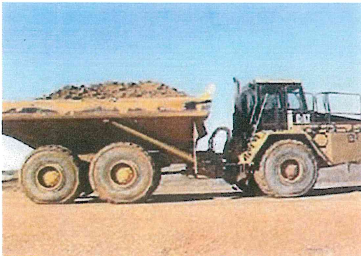
Cover soil hauled by ADT haul truck. Average load 30 yards.
