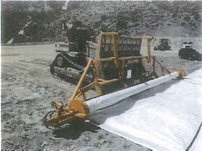
Deployment of tarpomastic tarp
