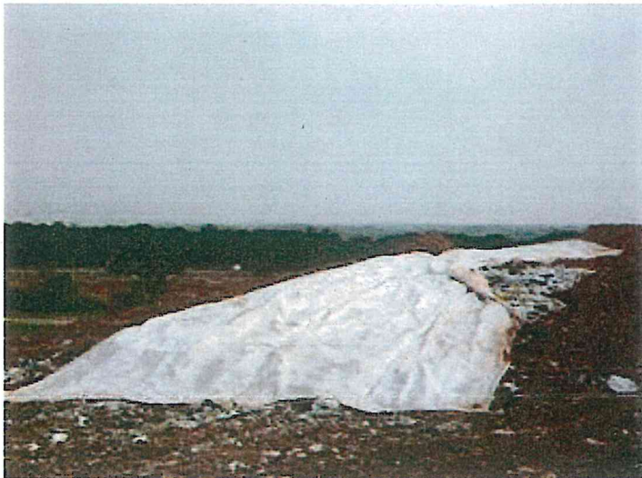
Landfill active area with tarp deployed and waste underneath tarp
