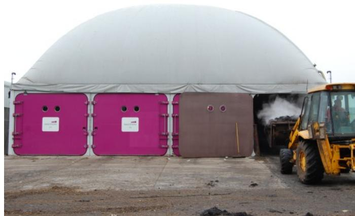
The AD facility stores methane gas in an inflatable storage bladder above the digestion chambers.
