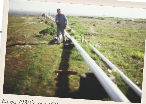
Early 1980's landfill gas collection system
