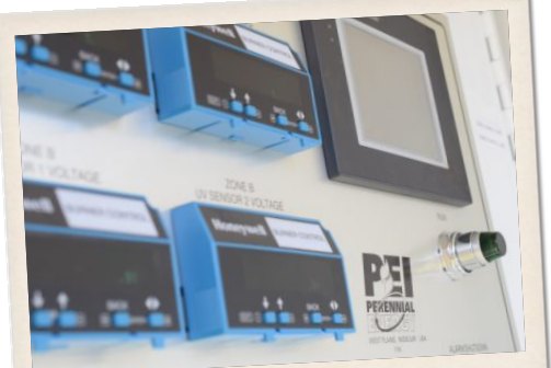
Today the Landfill Gas Project produces 5 megawatts of electricity
