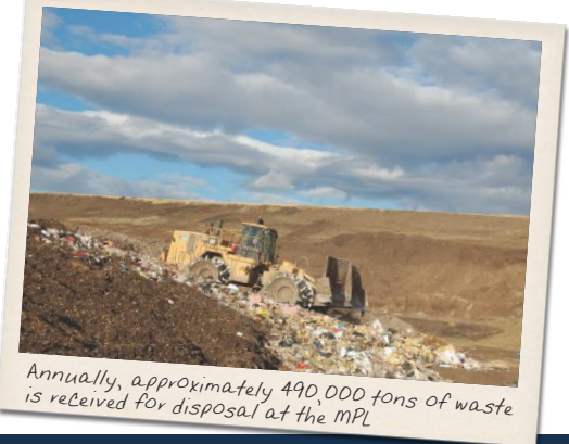
Board opens new landfill module, 2013
