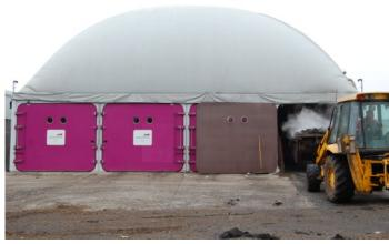
The AD facility stores methane gas in an inflatable storage bladder above the digestion chambers.
