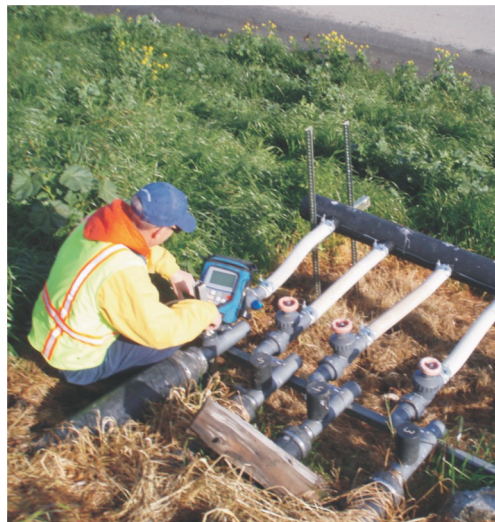
Staff measure landfill gas flow, composition and check for potential gas migration.
